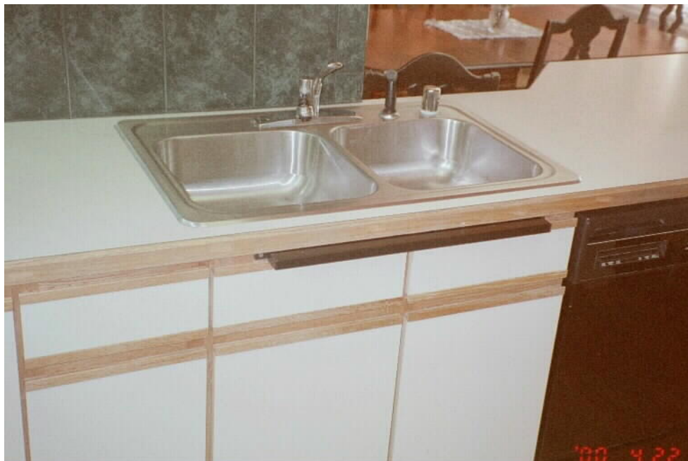
Figure 5.6 Hands free faucet controller (black bar under counter sill)
